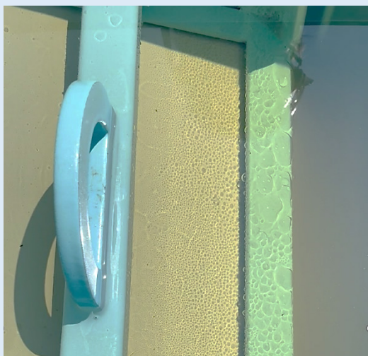
Dielectric fluid floating on water in an oil-water separator
