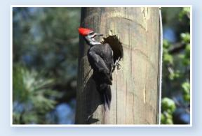
Woodpeckers can cause significant damage to wood poles in a short amount of time
