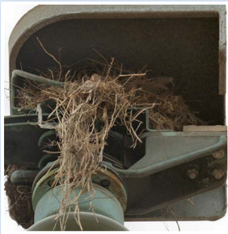
House Sparrow nest constructed on top of a gang-operated switch
